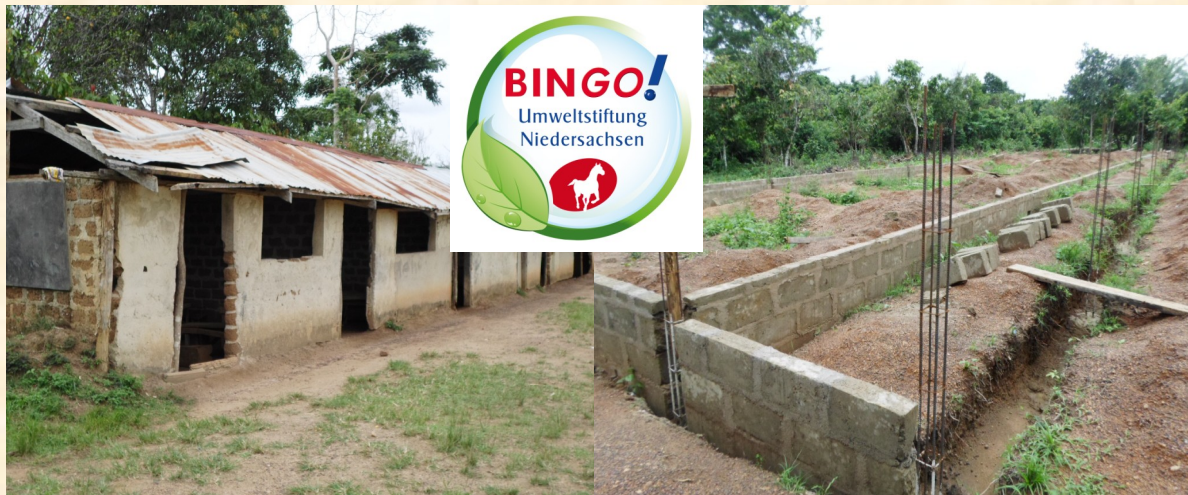
The picture on left shows the state of the school building which necessitated the construction of a new block. The picture on right shows the new building under construction.
