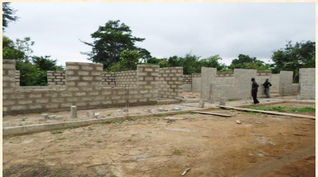
The school building in progress
