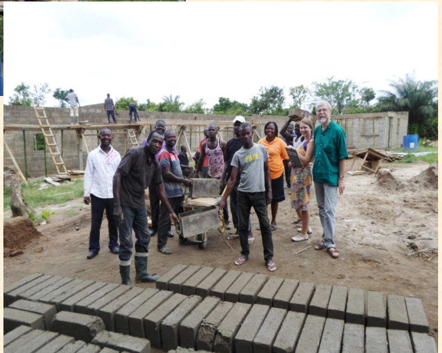
Work on the Anthony School project is steadily on course
