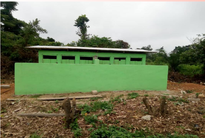
Toilet Facility at Anthony Completed
