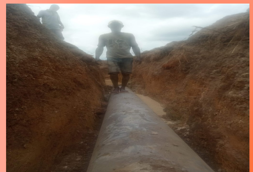
Laying of underground pipes in the main canals
