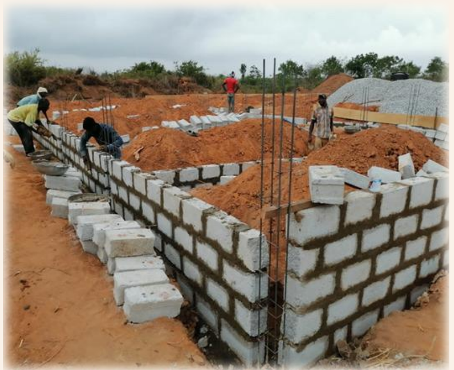
WORKERS LAYING THE FOUNDATION
